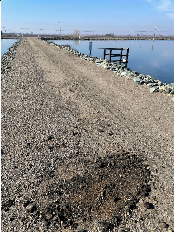
Photo 3 (left): View looking west near Boring B-2. Raveling and asphalt deteriorating.
