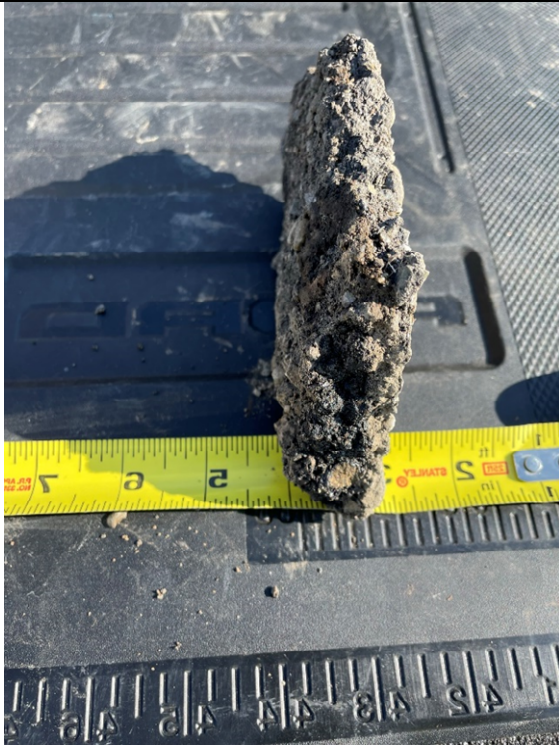
Photo 1: Typical asphalt concrete thickness
