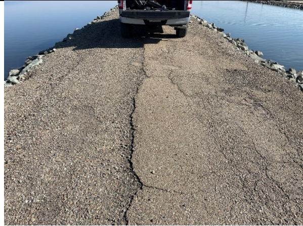
Photo 3 (left): View looking west near Boring B-2. Raveling and asphalt deteriorating.
